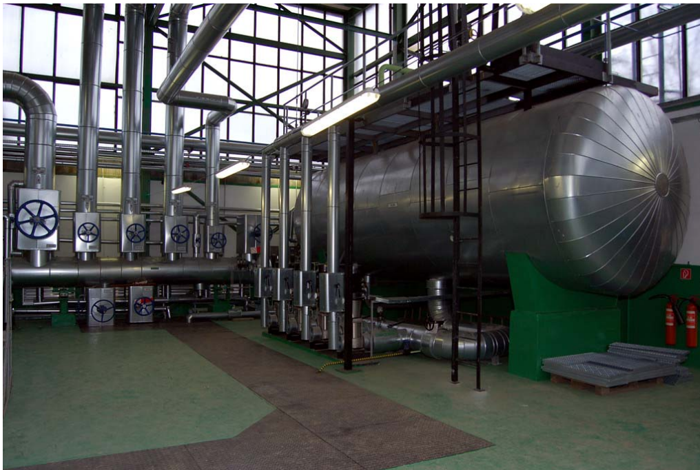
Picture No. 25 V1 Nuclear Power Plant - Reconstructed auxiliary boiler room
