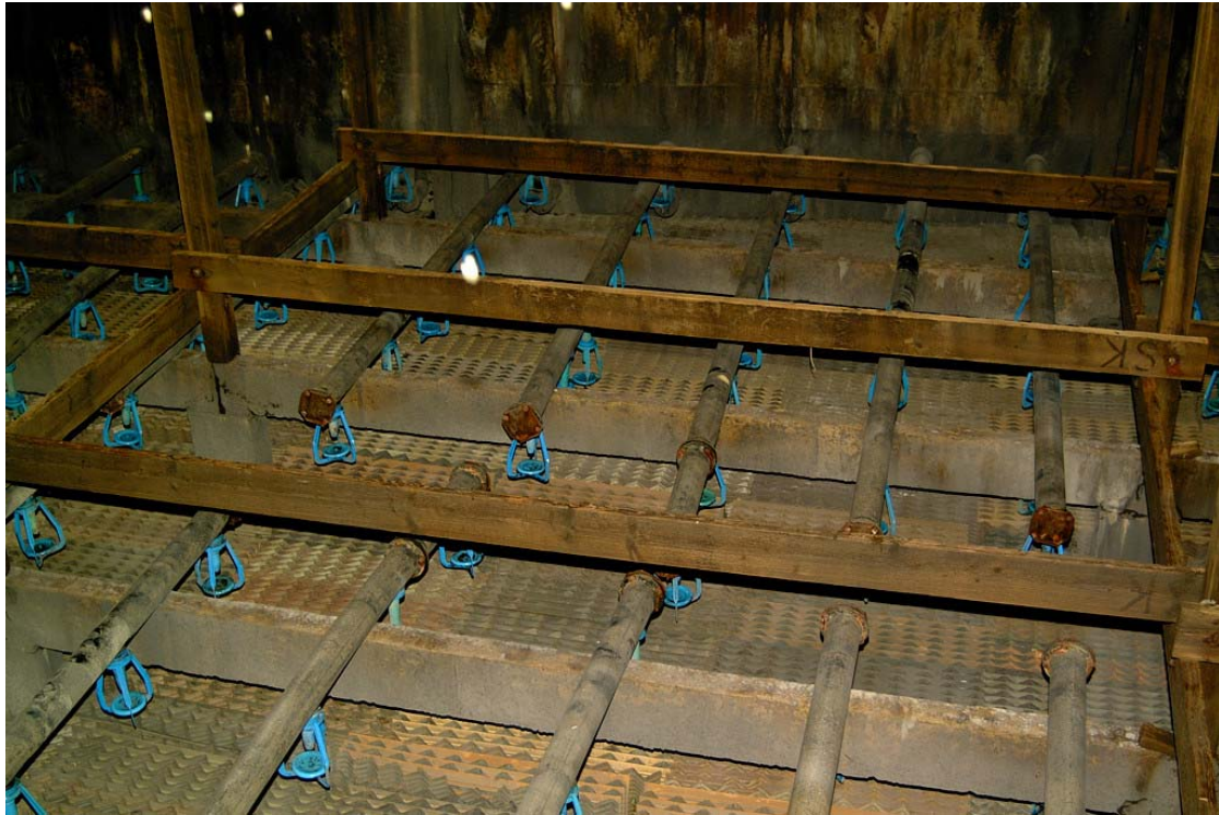
Picture No. 3 V1 Nuclear Power Plant - Spraying jets in tower
