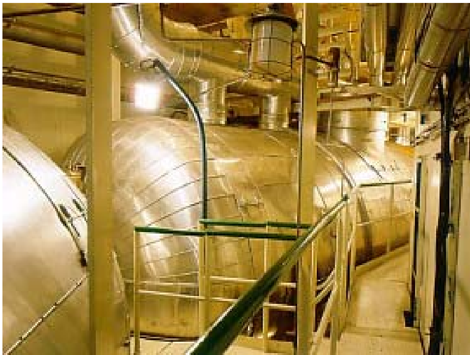
Picture No. 18 V1 Nuclear Power Plant - Steam generators of WWER 440
