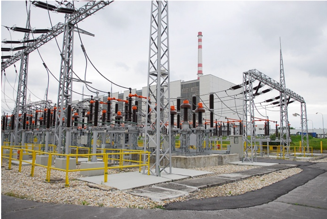
Picture No. 23 Switchyard Tr 110kV - NPP V1 (will be reconstructed)
