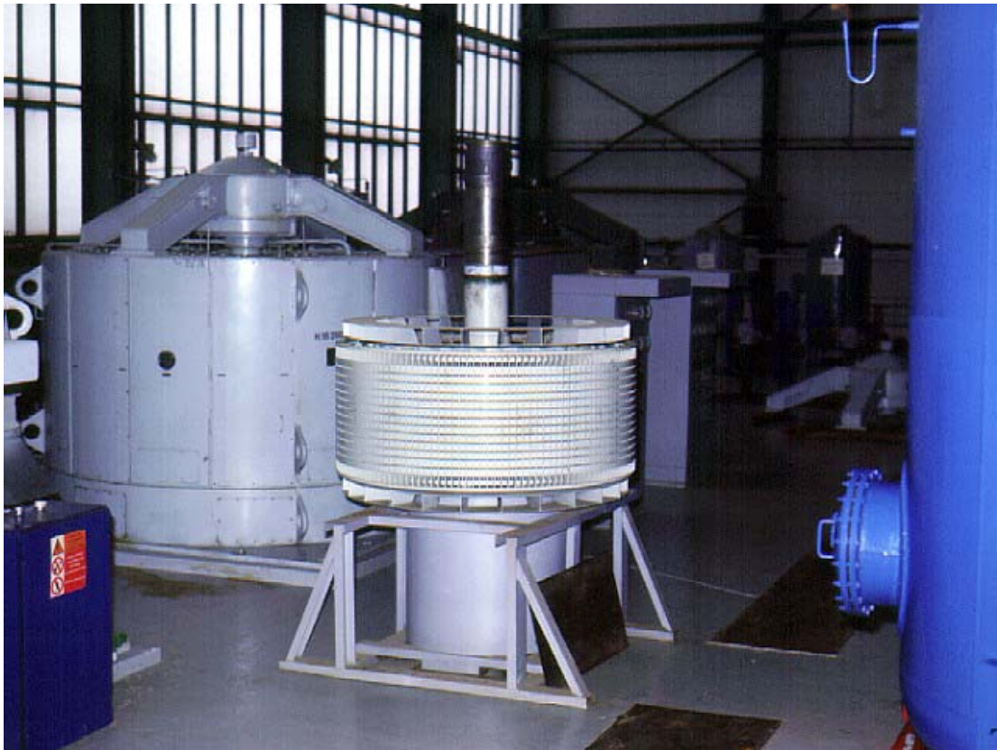
Picture No. 5 V1 Nuclear Power Plant - Cooling water pumps in building of pump station
