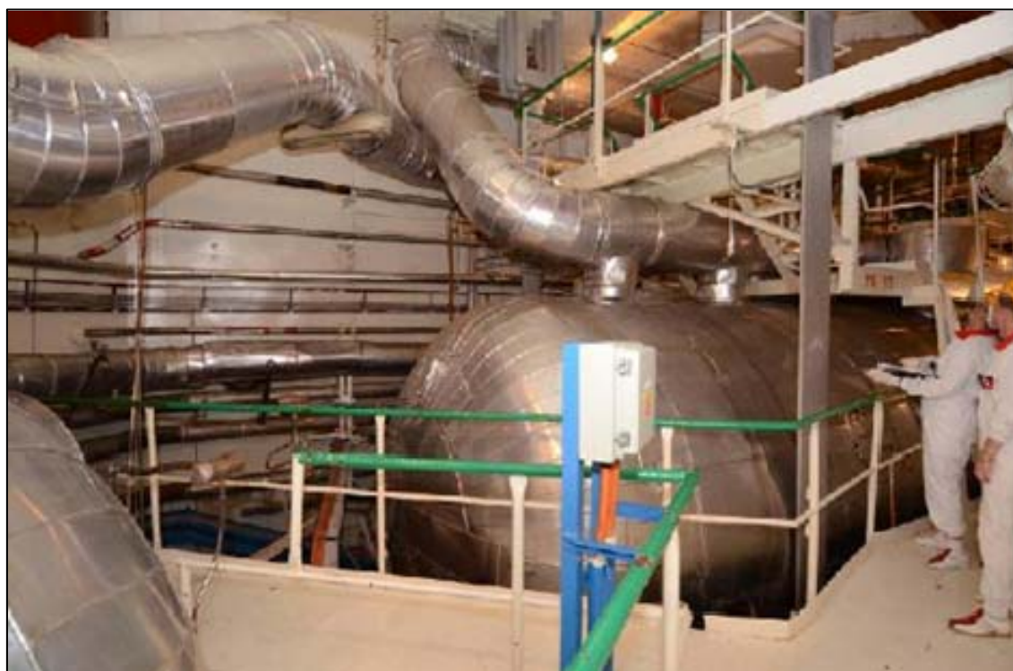
Graph No. 24. SGs Insulation shell
