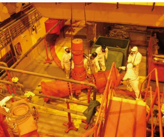
Decontamination of turbocharger of charging machine
