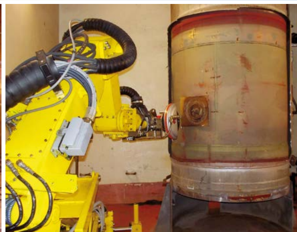
Fragmentation of heavy water evaporator with remote controlled manipulator
