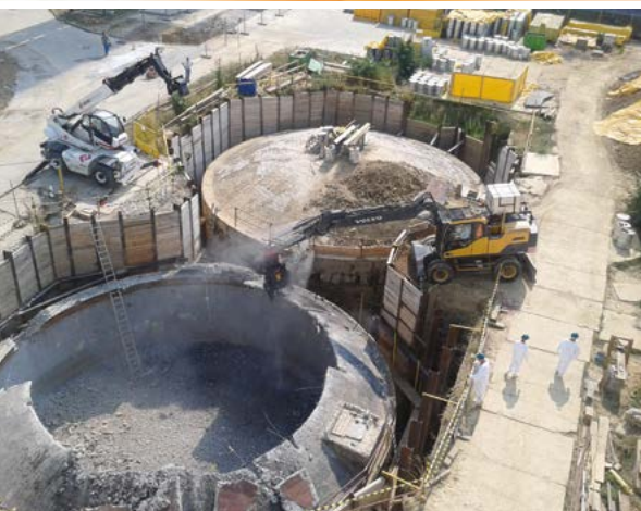
Decommissioning of LRAW external storage tanks
