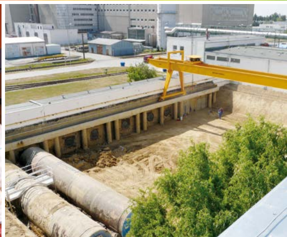
Decommissioning of CO 2 gasholders
